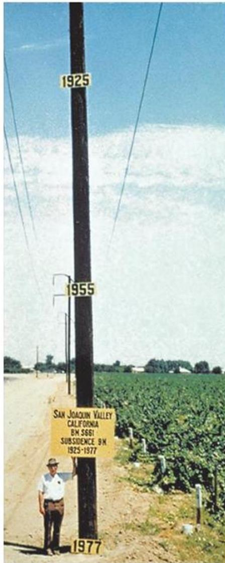
Figure 1. Approximate location of maximum measured subsidence (9 m) in the San Joaquin Valley, California (1925–77) attributed to aquifer-system compaction caused by groundwater abstraction. Signs on pole (1925, 1955) are positioned at approximate former elevations of land surface. Pictured is Dr. J.F. Poland; photograph by R.L. Ireland, USGS, ca. 1977.
